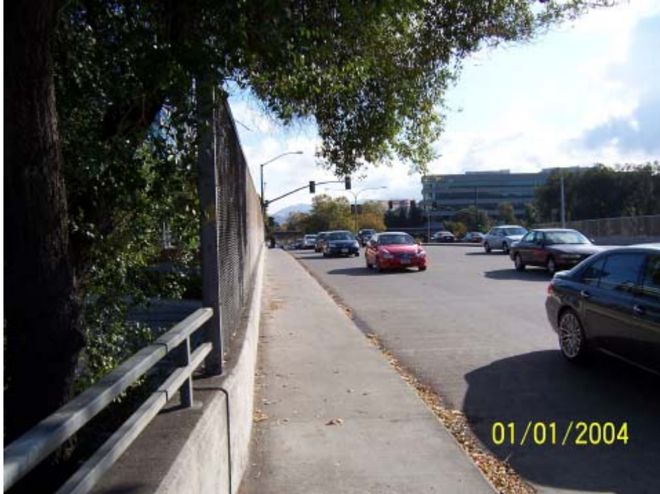
North Side of Treat Boulevard/I-68o Over-Crossing Looking East Toward Contra Costa Centre
