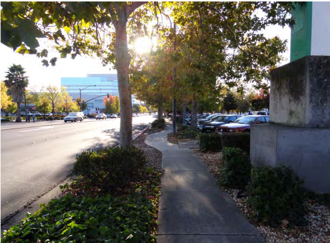
12. North-side Willow Pass Road: Proposed improvements include widening the existing sidewalk to 8' where feasible, replacing the meandering style through streetlight poles & landscaping and repairing trip hazards due to tree roots.
