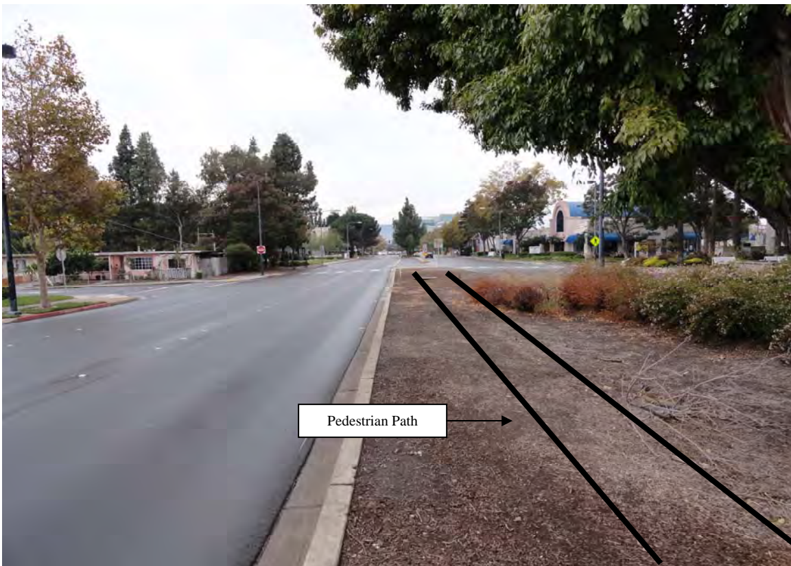
4. Island Median @ Clayton Rd/Sutter St: Proposed improvements include new Pedestrian Path connection from pedestrian refuge @ traffic signal to new crosswalk location.
