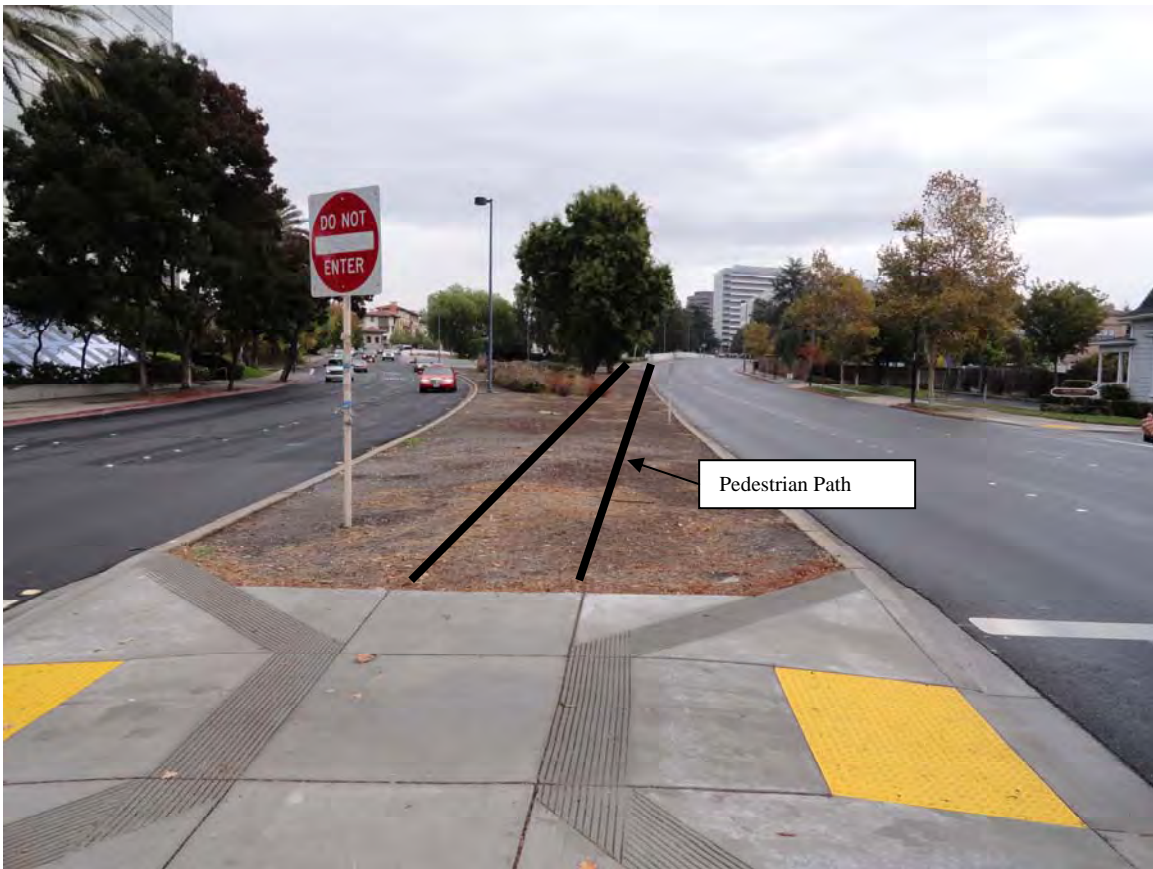
3. Island Median @ Clayton Rd/Sutter St: Proposed improvements include new Pedestrian Path connection from pedestrian refuge @ traffic signal, to new crosswalk location.
