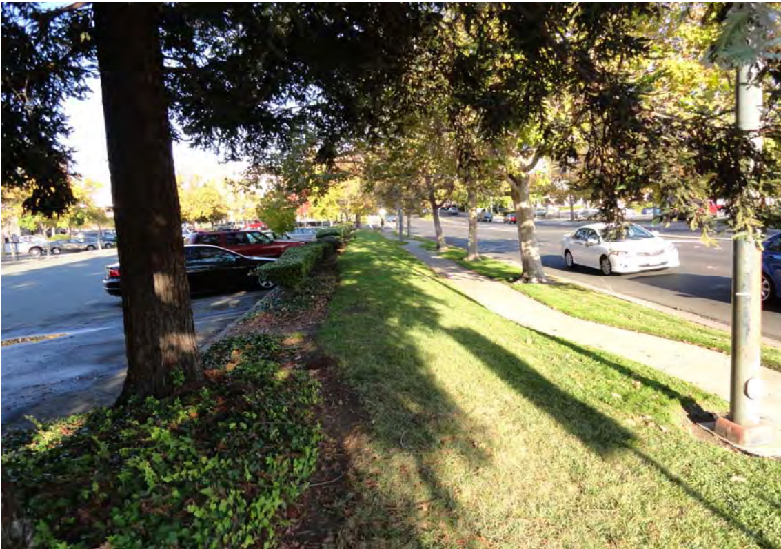
11. North-side Willow Pass Road: Proposed improvements include widening the sidewalk to 8' where feasible and evening out grade issues, including installation of pedestrian seatwalls where possible.
