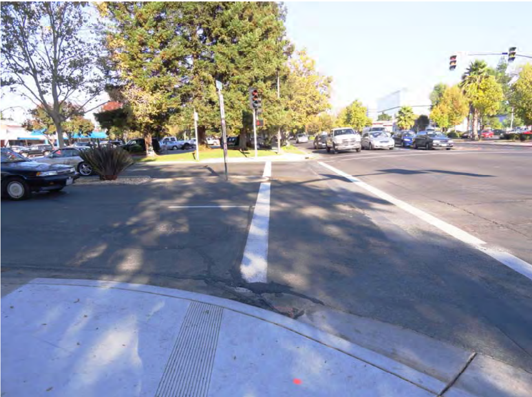
13. North-side Willow Pass Road @ Fry Way: Proposed improvements include replacing existing crosswalks with ADA-compliant, high-visibility color concrete crosswalks.
