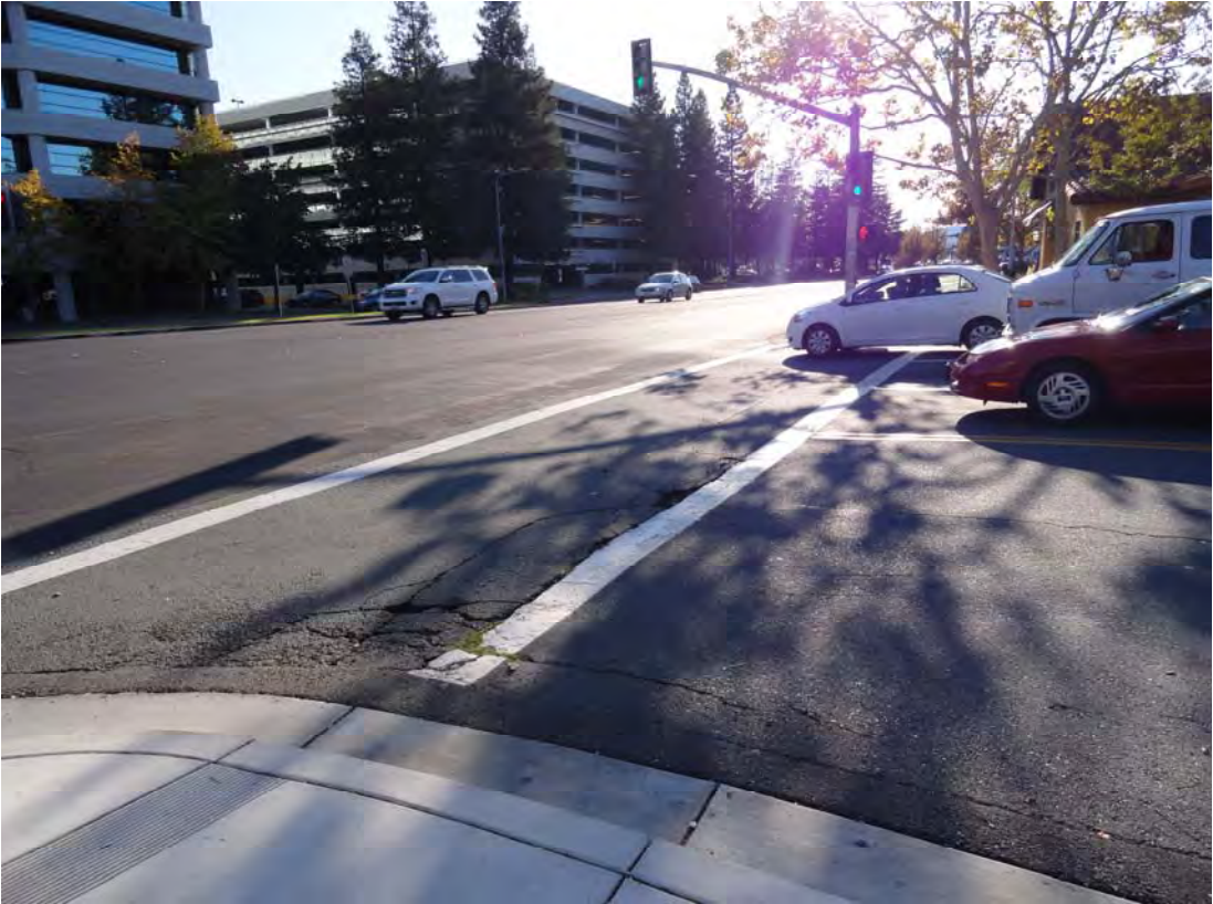
14. North-side Willow Pass Road @ Gateway Blvd: Proposed improvements include replacing existing crosswalks with ADA-compliant, high-visibility color concrete crosswalks.
