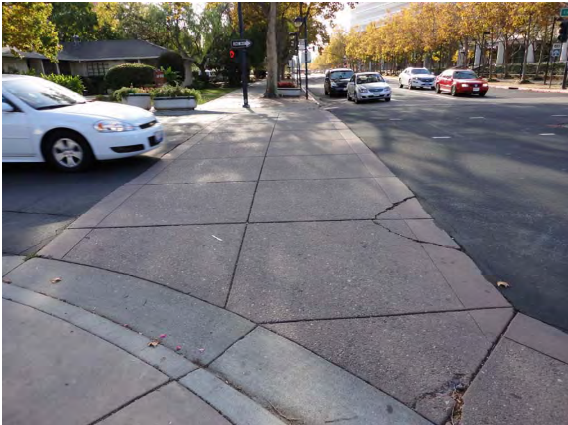
8. Concord Blvd @ Grant St: Proposed improvements include replacing existing pothole & crack-ridden crosswalks with ADA-compliant, high-visibility color concrete crosswalks.
