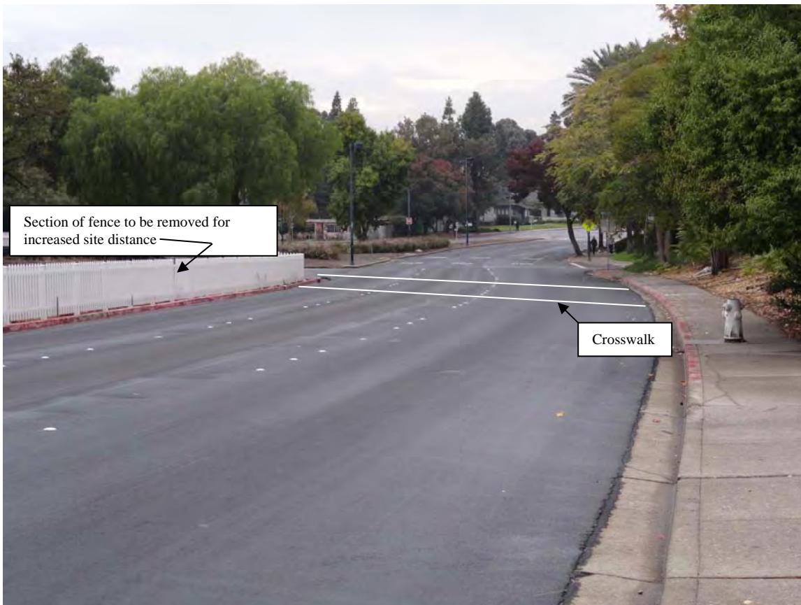
6. West-bound on Concord Blvd (near Mira Vista Terrace): Install new crosswalk and remove section of decorative fence
