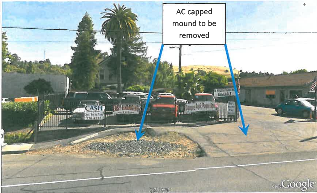
3782 Pacheco Boulevard, AC capped mound to be removed
