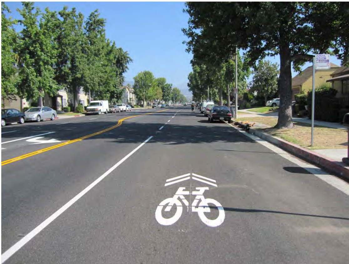
16. Grant St (BART station, through Downtown to Adobe St) and Salvio St (East St to Market St): Proposed improvements include installation of a Class 3 bike route throughout the Downtown area with signage and 8 bike lockers for safe storage.
